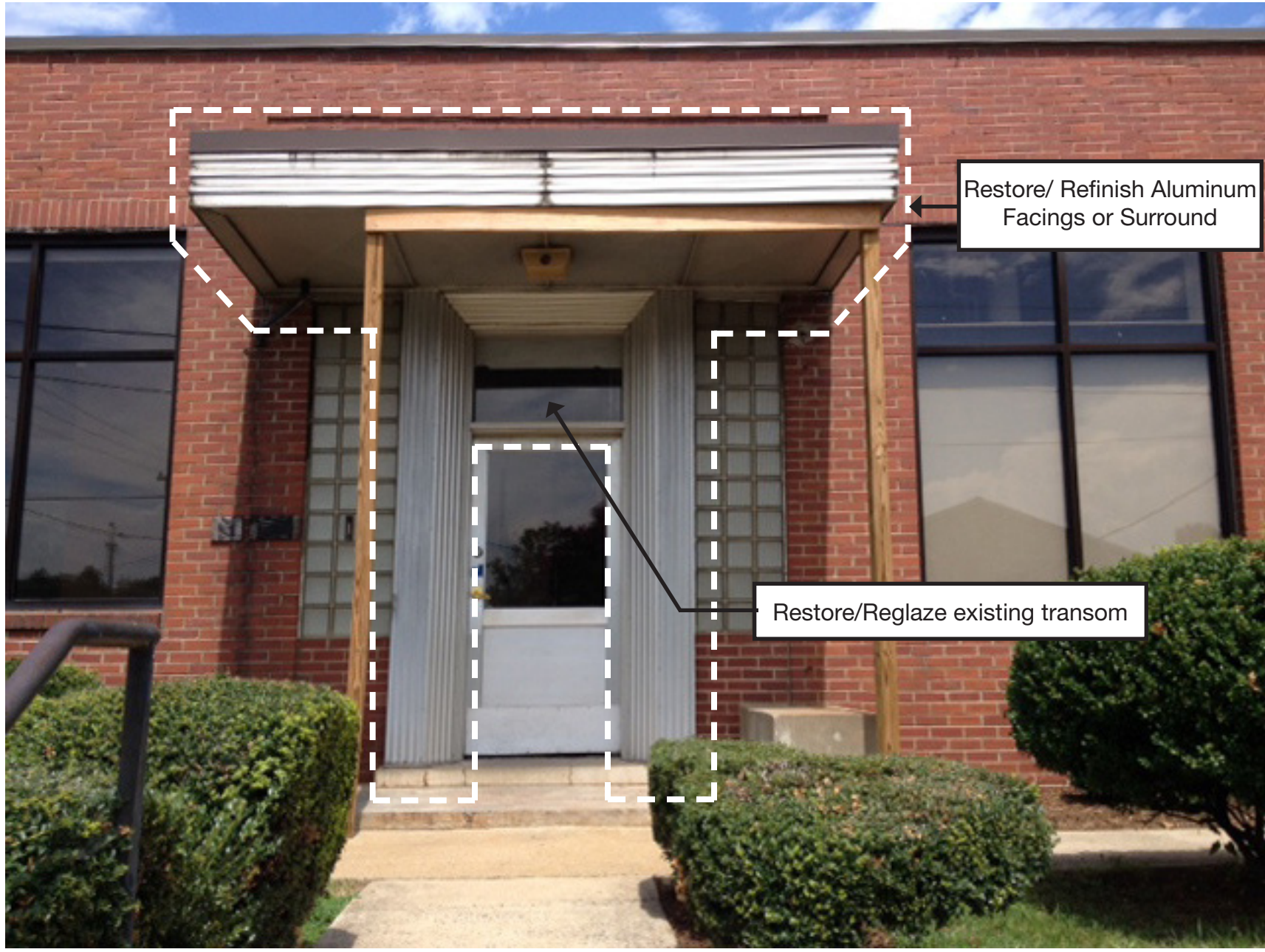
Existing Condition of Entry Door
