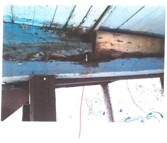
Rotten Floor Joists under Weight bearing wall of addition
