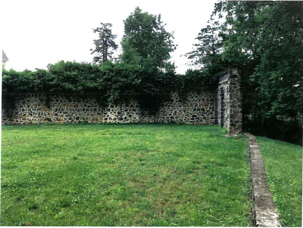
East edge of proposed section to be demolished
