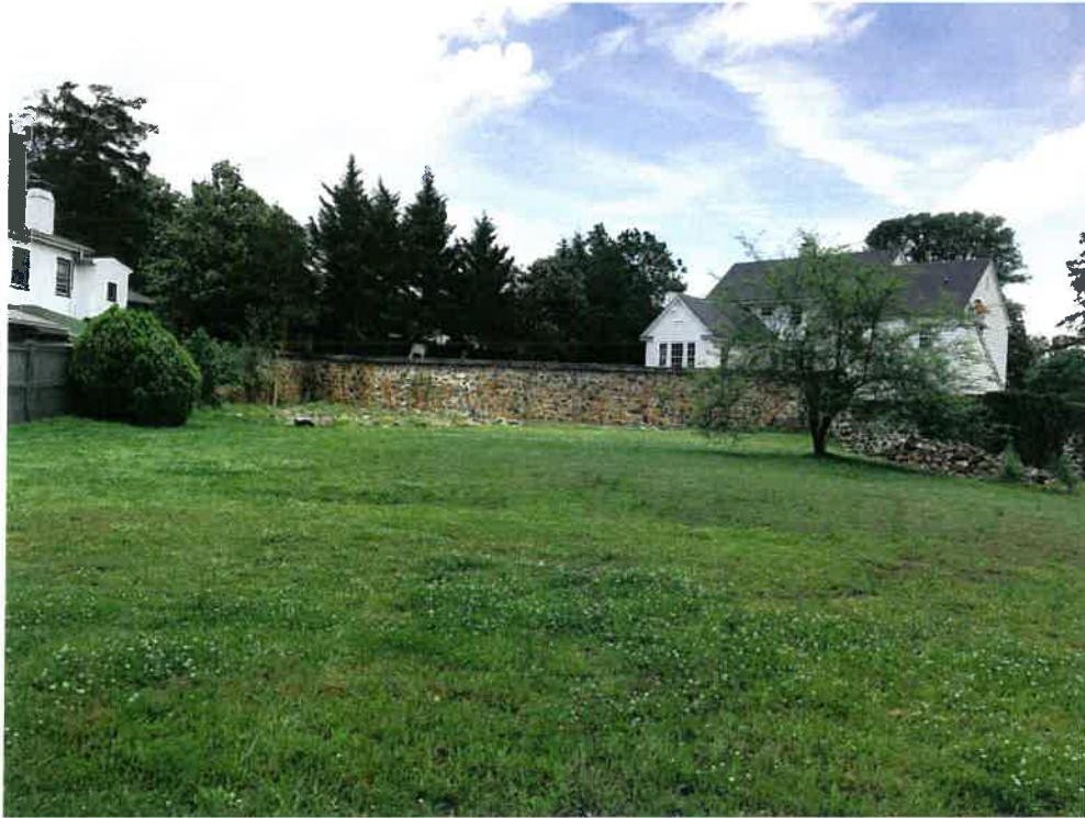
Proposed section to be maintained: see clear step down and change in construction method between areas to be maintained and demolished
