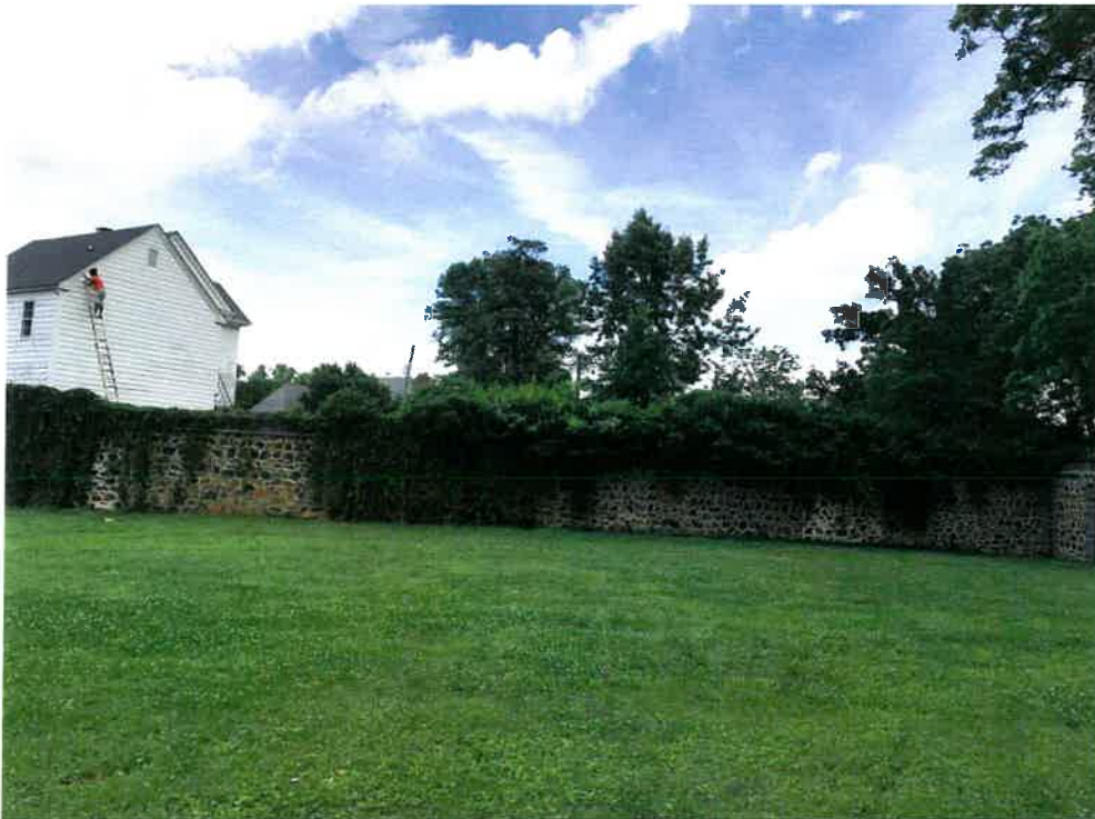
Area to be demolished
