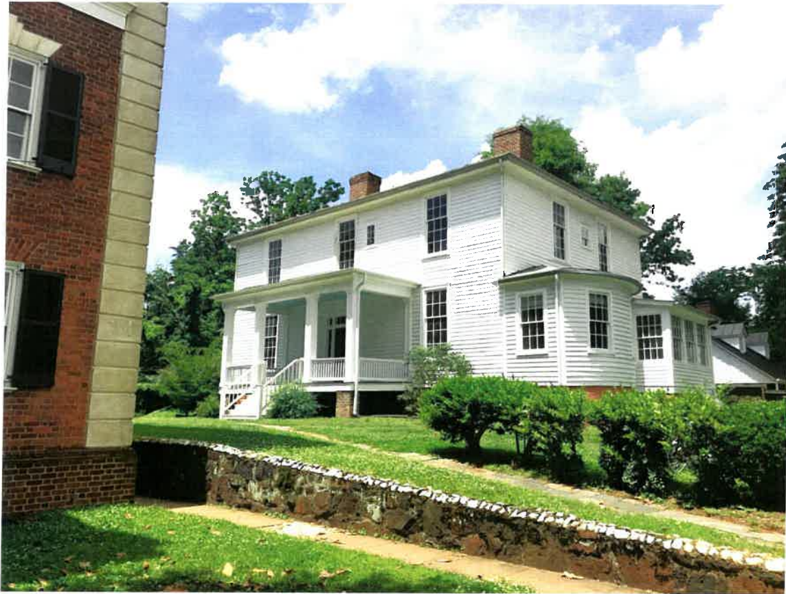
View of the Front of the House showing Apartment Building Corner
