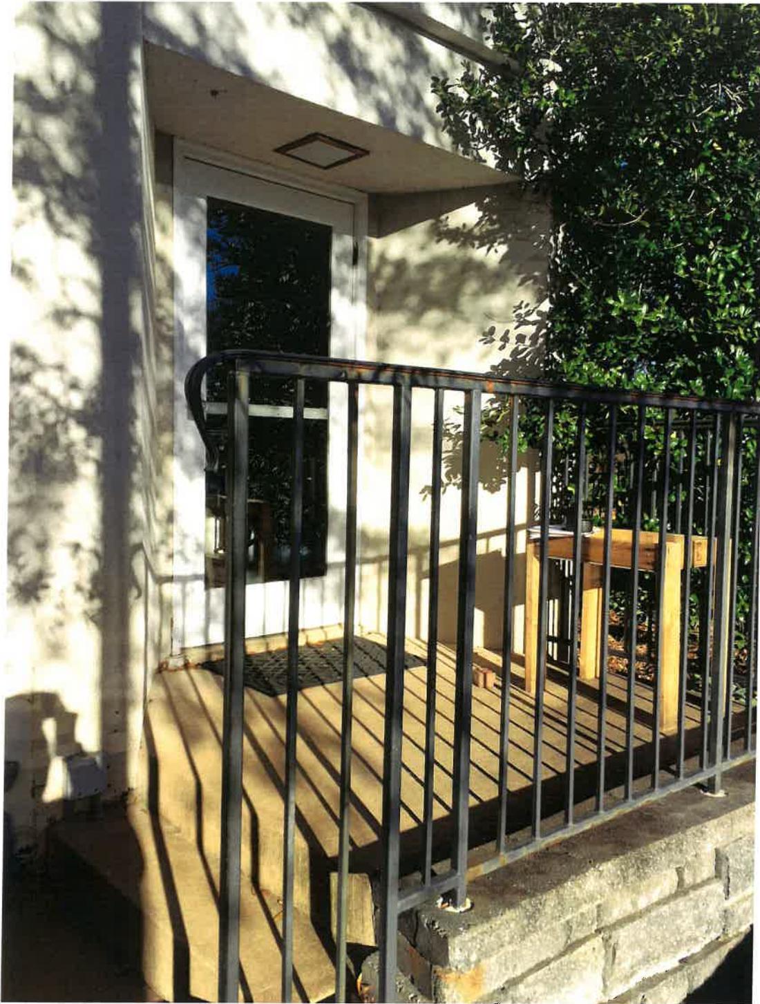
VIEW OF STAIR TOWER ENTRANCE
