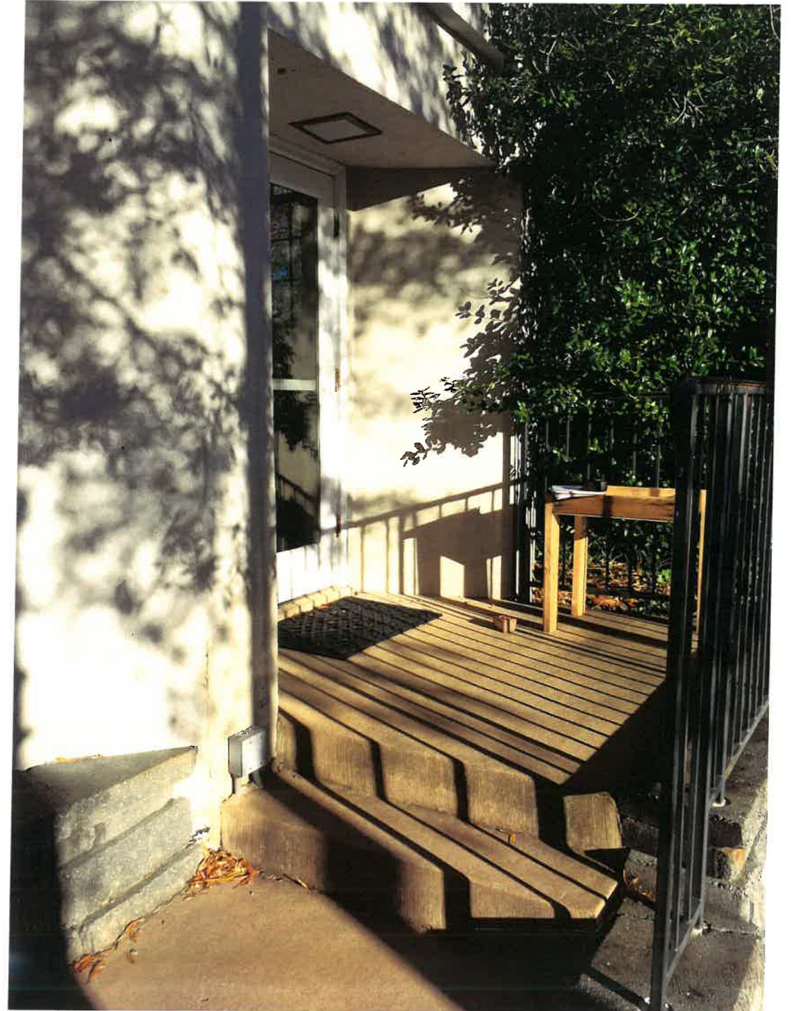
VIEW OF STAIR TOWER ENTRANCE
