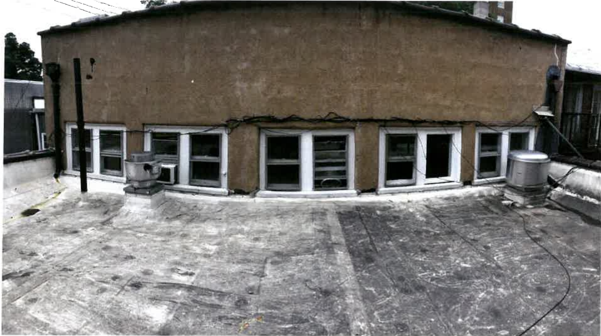
2 nd Floor Rear Windows
