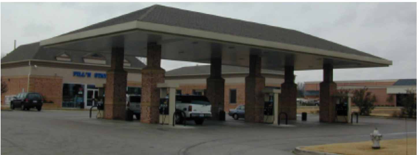
The piers supporting this canopy are clad in the same brick as the surrounding buildings and numerous recessed lights provide adequate lighting.
