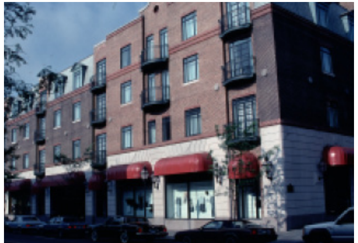
This Charleston, South Carolina hotel uses a decorative stone base, two colors of bricks, a shingle mansard roof, iron balconies and colorful awnings to divide up this monolithic structure.
