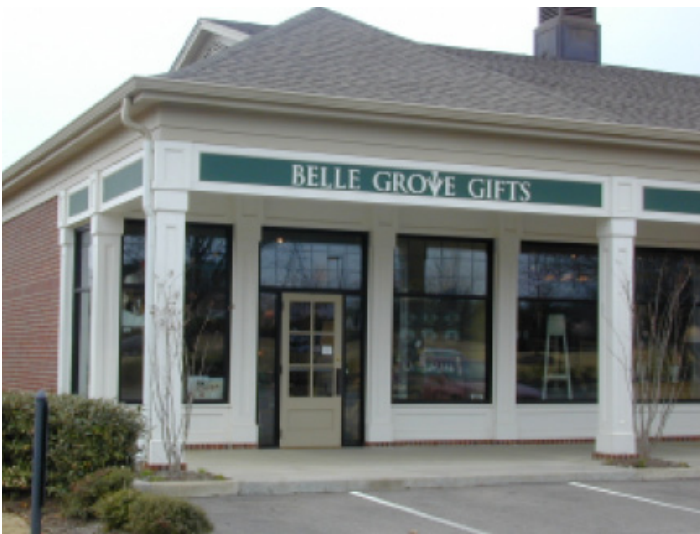
This storefront design is well detailed with transoms and an integrated sign band.
