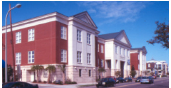
This library facade has three projecting classical bays to reduce its mass and parking is contained within the first floor of the structure.
