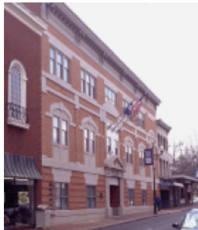
This facade has a traditional decorative cornice along with cast stone and masonry to divide up its large mass.
