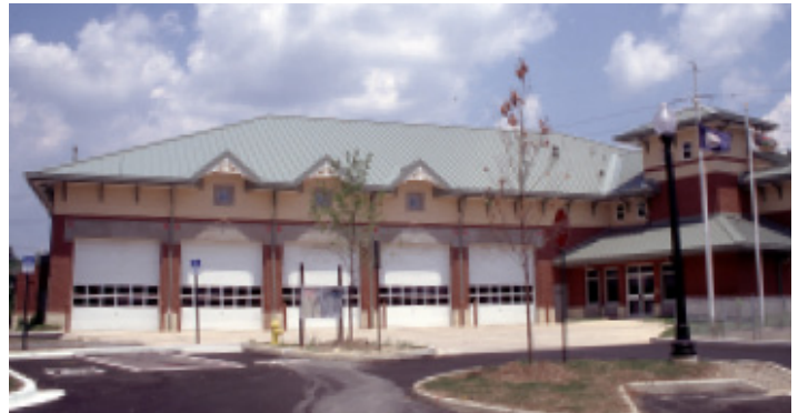
Several types of masonry along with a metal roof and decorative details create the distinctive design of this fire station.
