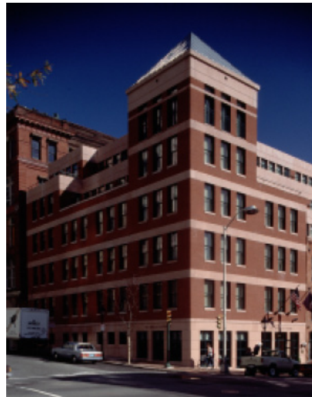
This stepped roof corner tower serves as a gateway feature and also helps screen the stepped back upper floors of this Richmond hotel.
