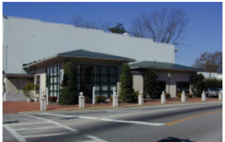
In this example, a former service station has been redesigned to serve as the town's chamber of commerce.
