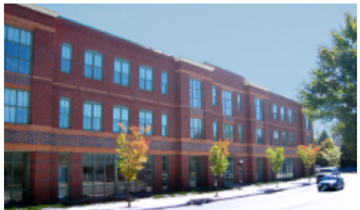
The use of vertical bay divisions and horizontal bands of masonry patterns visually reduce the mass of this office building.
