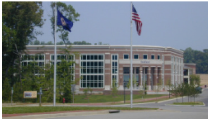
This new bank is located along a corridor, is buffered by a wooded strip and has a modulated facade to reduce its scale.
