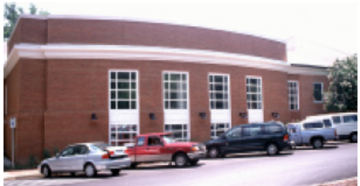
The bow-shaped addition to a community center continues the brick material, as well as the classical cornice line, while introducing larger more contemporary-sized windows.
