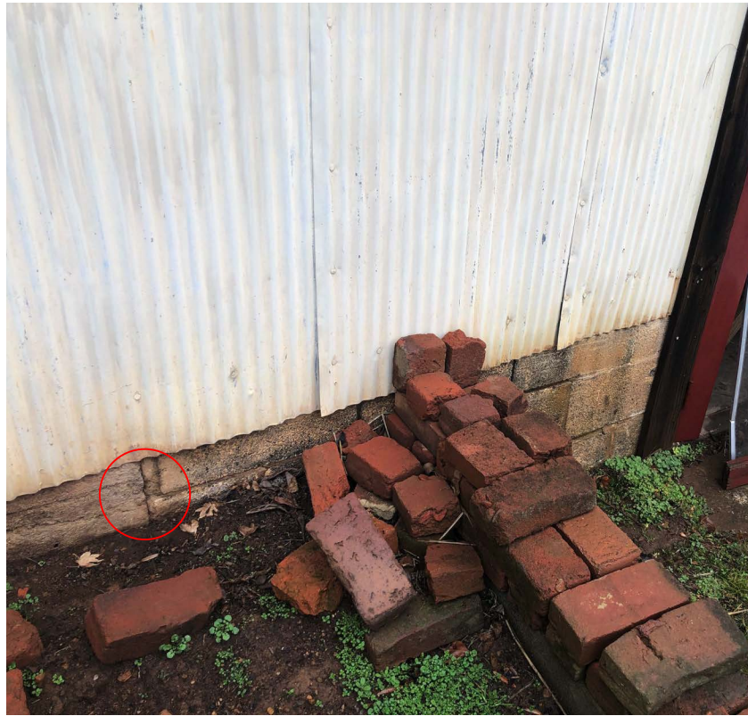
FOUNDATION TRANSITION: FOOTPRINT NOT ORIGINAL
