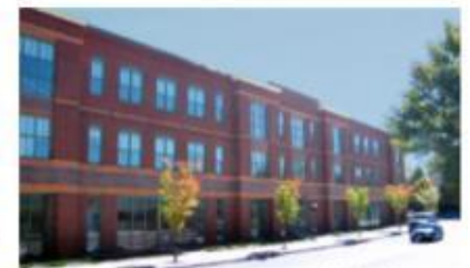
The use of vertical bay divisions and horizontal bands of masonry patterns visually reduce the mass of this office building.
