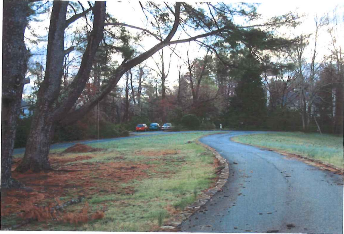
Figure 1: View along one-way exit lane towards site entrance
