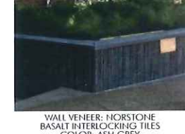
WALL VENEER: HORSTONE BASALT INTERLOCKING TILES COLOR: "ASH GREY"
