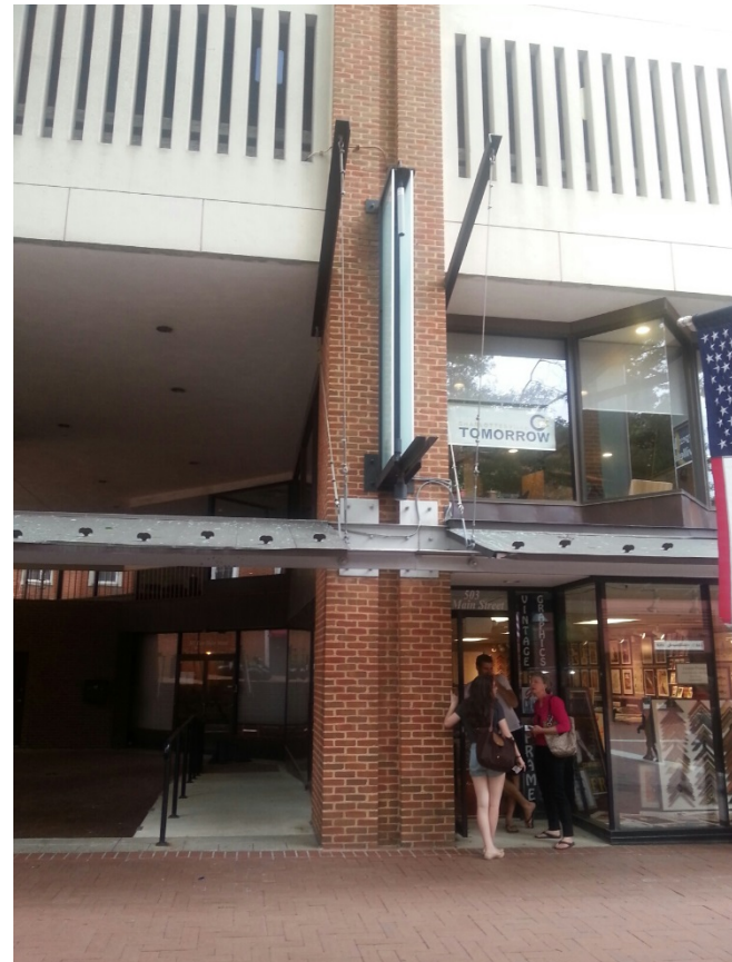
Cylindrical Antennas between Glass Light Fixture Panels
