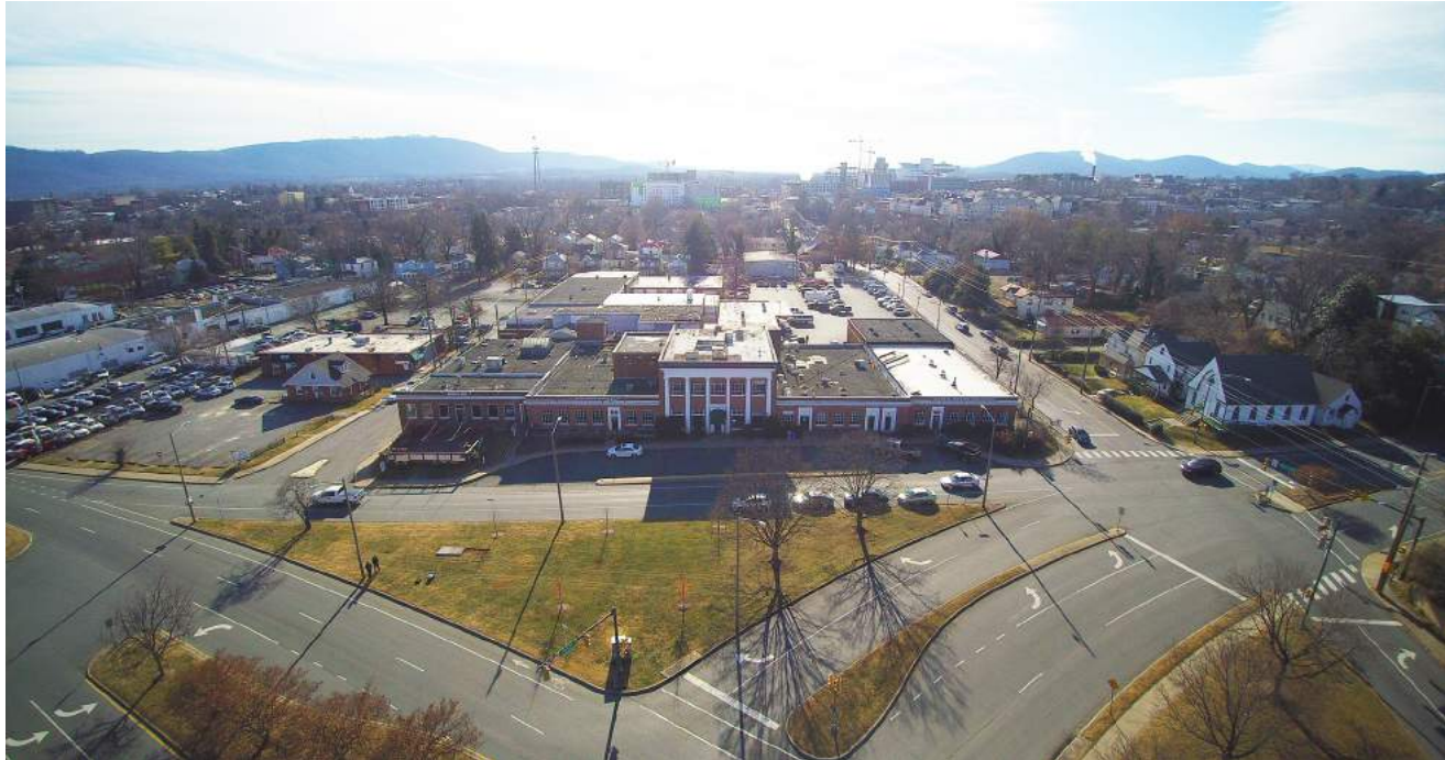
2. AERIAL VIEW OF THE SITE FROM THE NORTH
