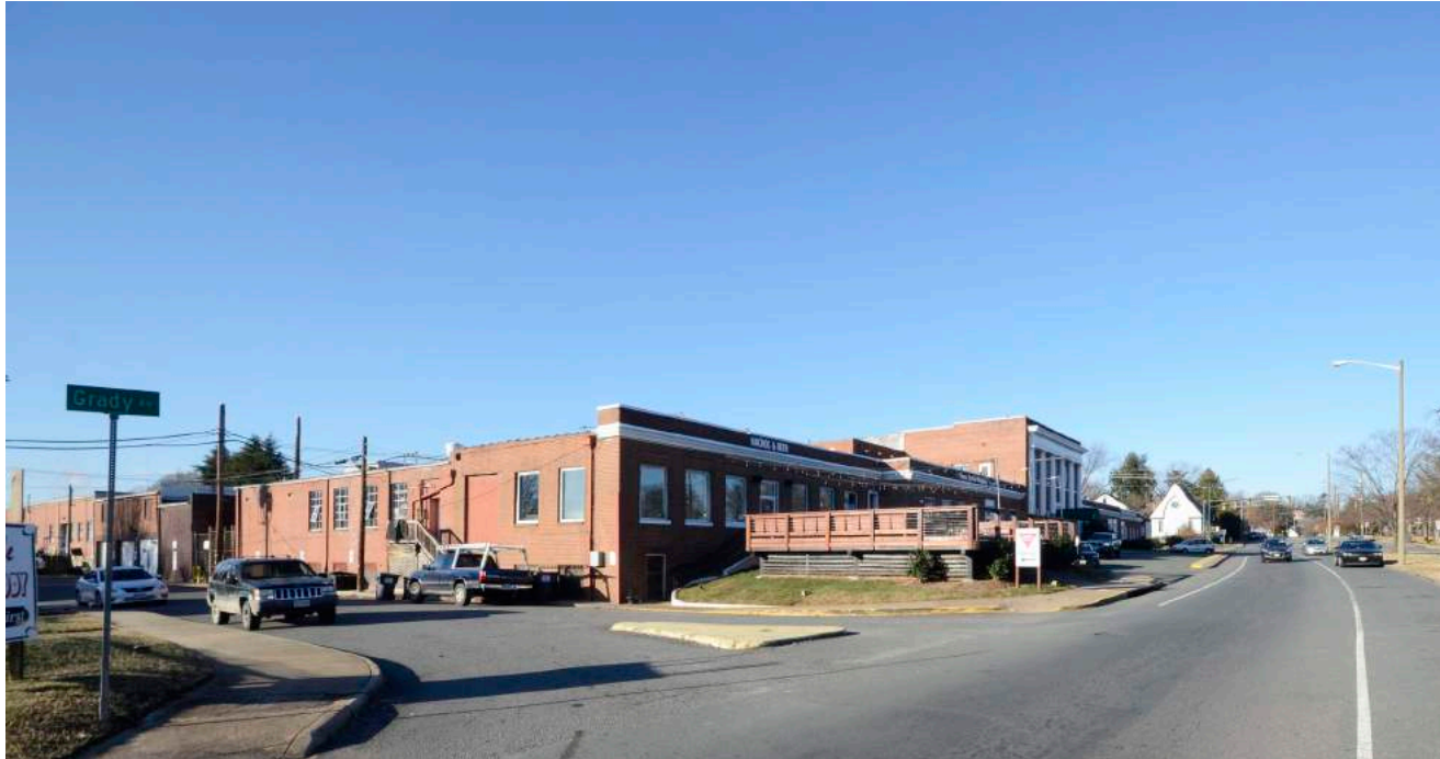
4. DAIRY BUILDING FROM GRADY AVENUE + WOOD STREET
