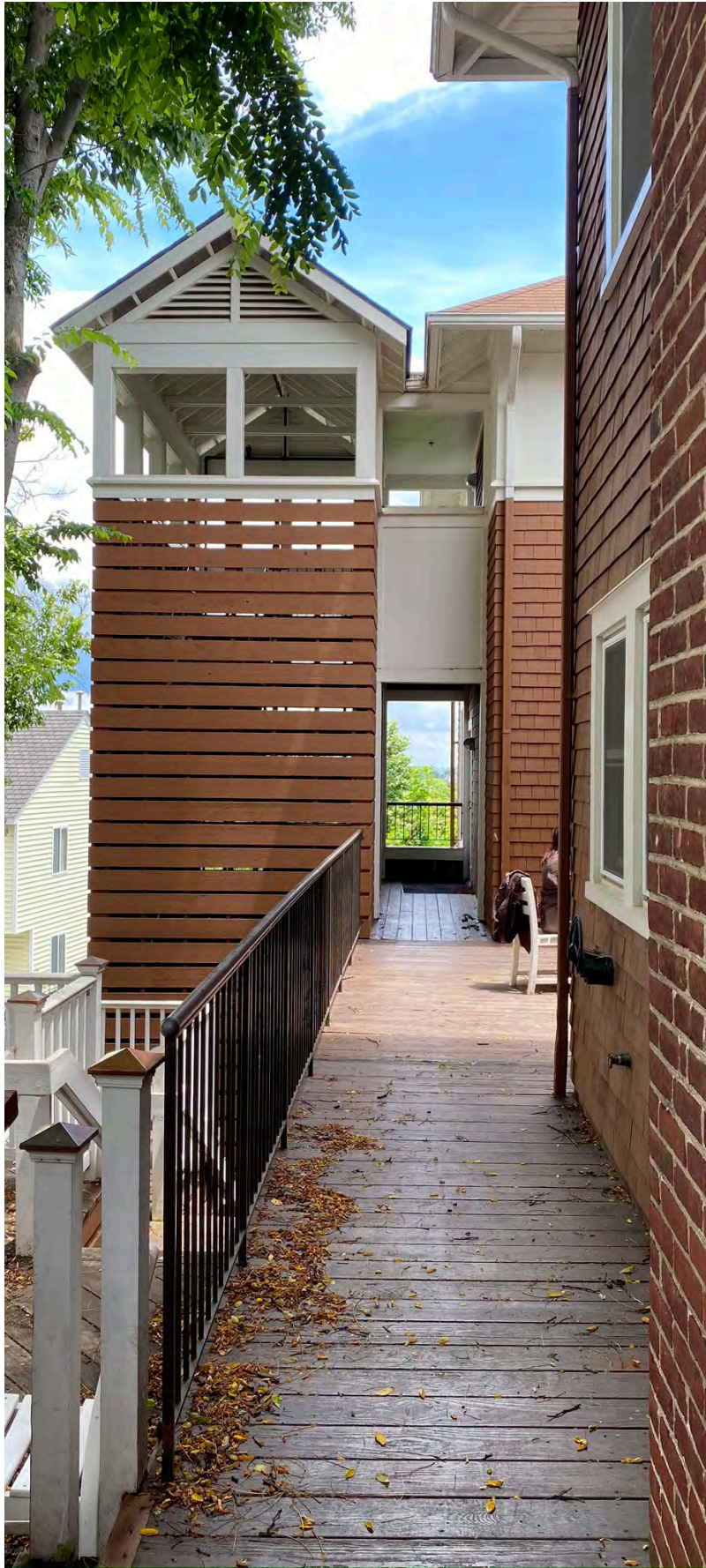
1. NORTH WALK LOOKING EAST
