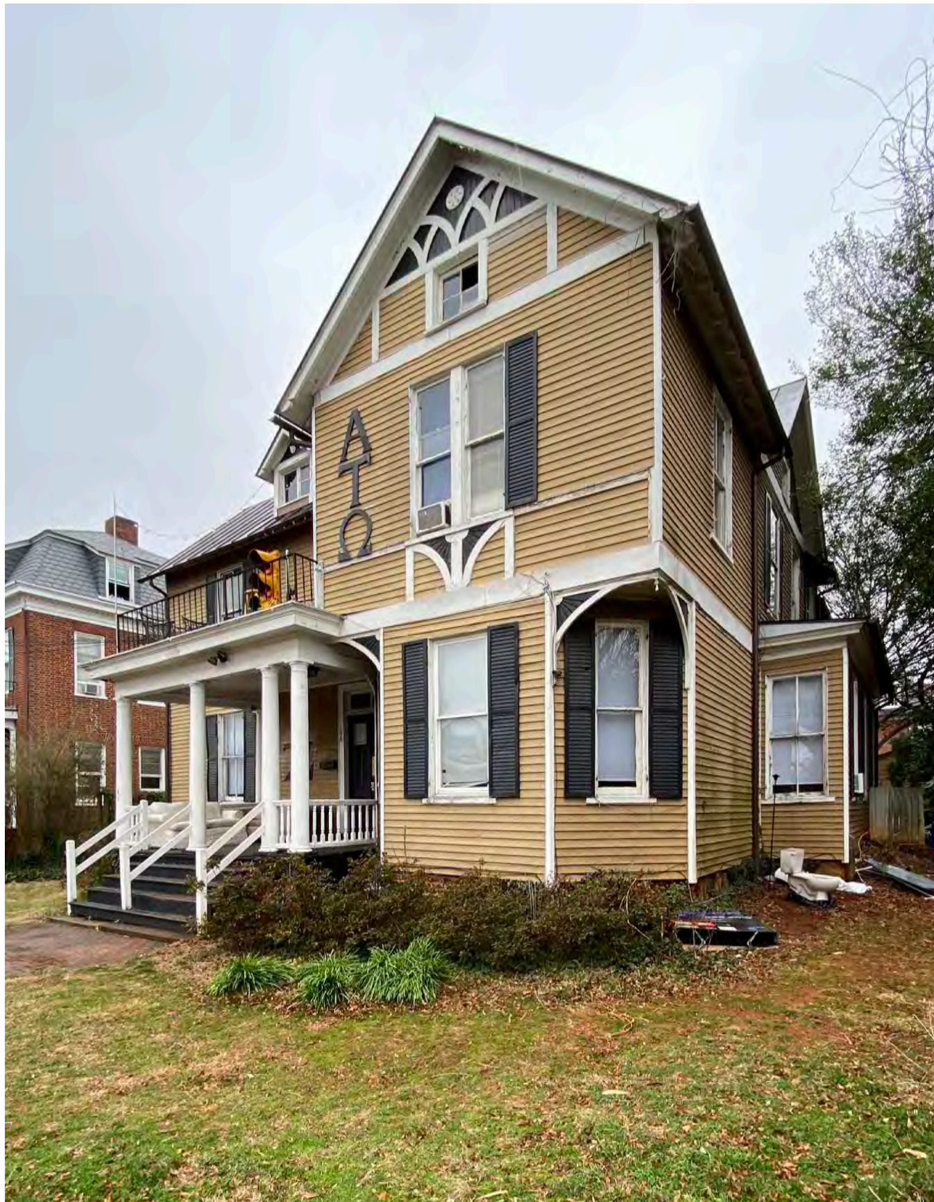
Existing Exterior N/E FRONT OF HOUSE
