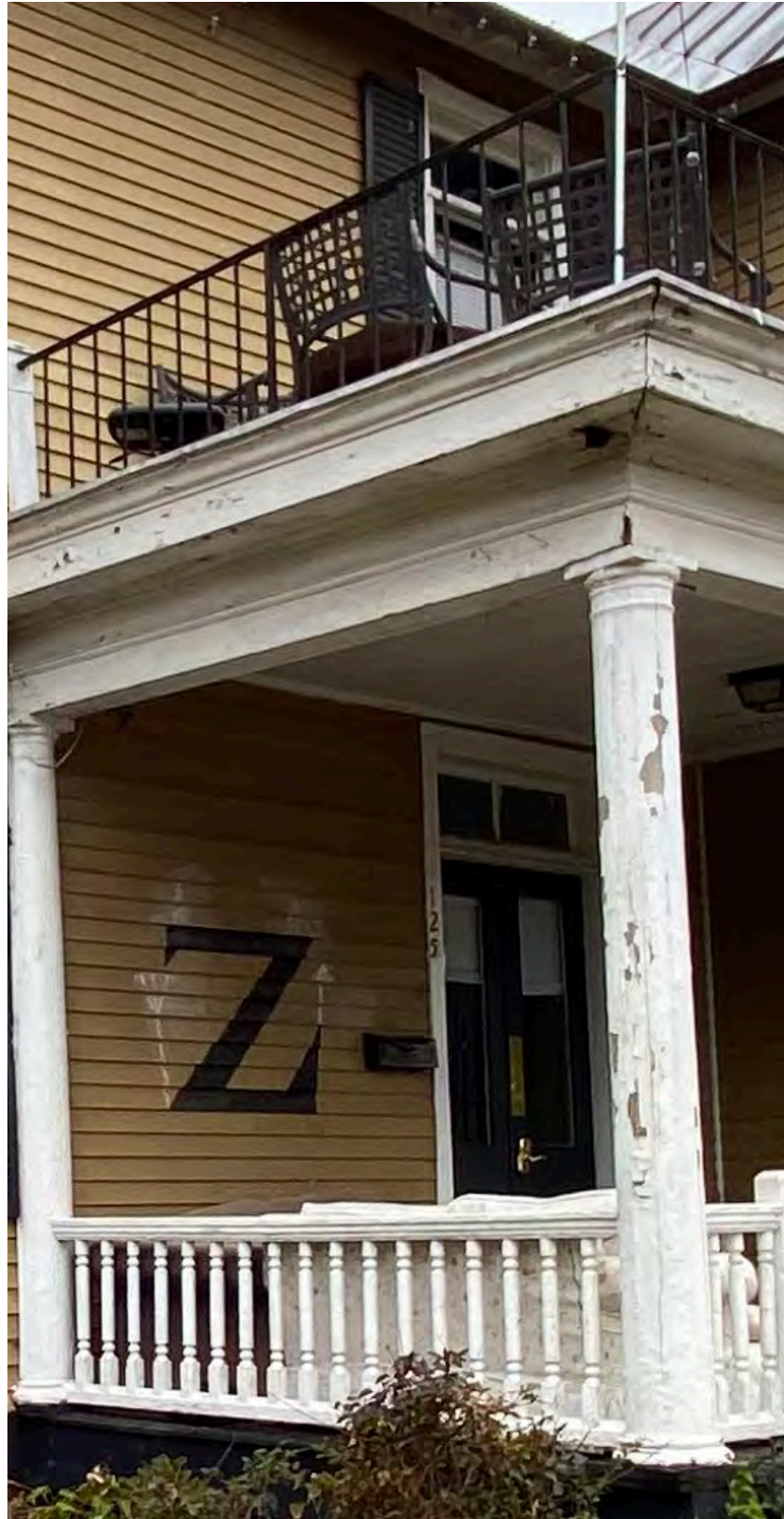
Existing FRONT PORCH
