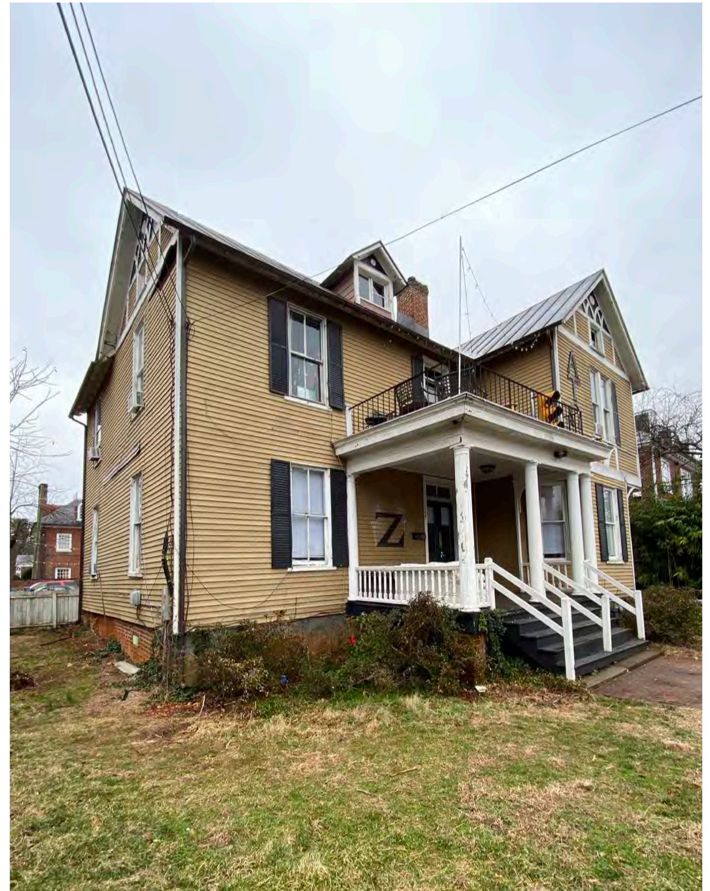
Existing Exterior S/E FRONT OF HOUSE
