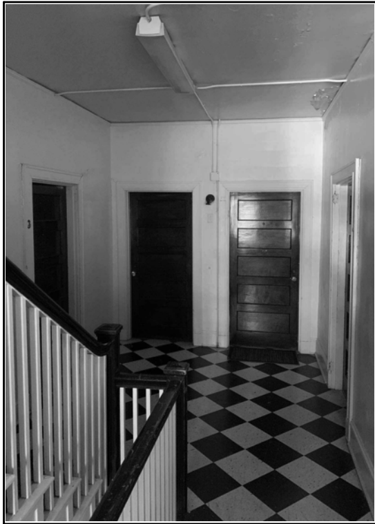
STAIR HALL WITH 4 ORIGINAL UNIT ENTRY DOORS PER FLOOR
