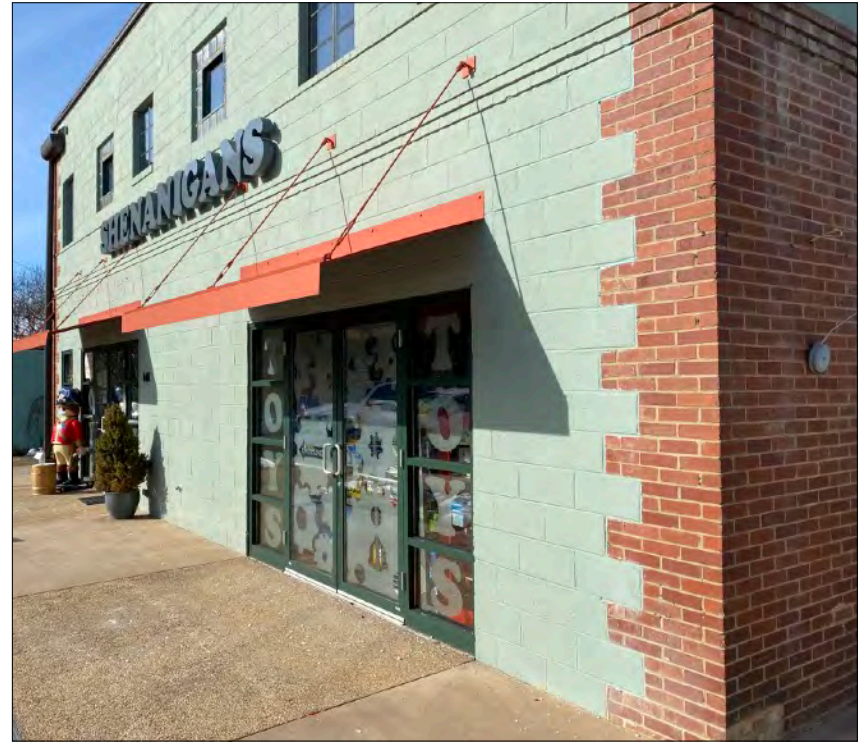
CANOPY- EXAMPLE, BOLT TO WALL AND CABLES
