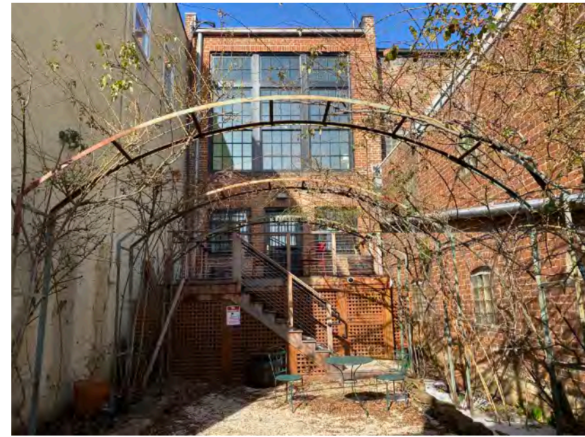
VIEW NORTH INTO A COURTYARD
