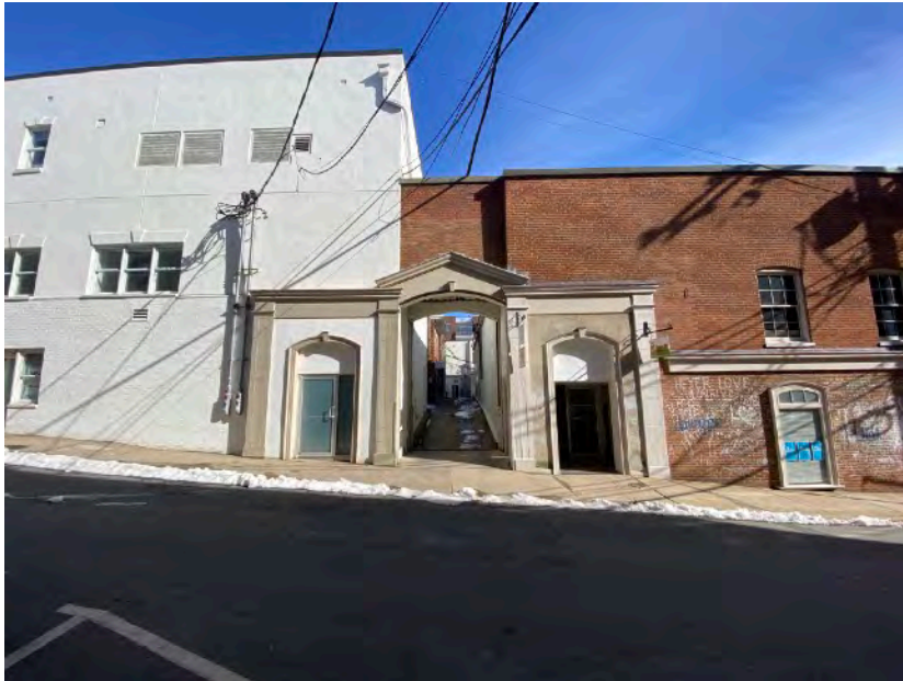
VIEW EAST FROM 4TH STRET NW
