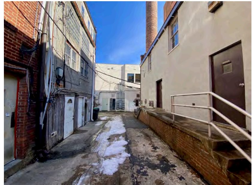
VIEW EAST AT FACADE
