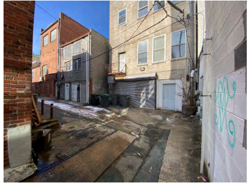
VIEW NORTHWEST AT FACADE
