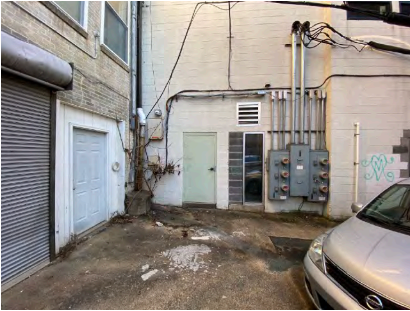
VIEW EAST PAST FACADE
