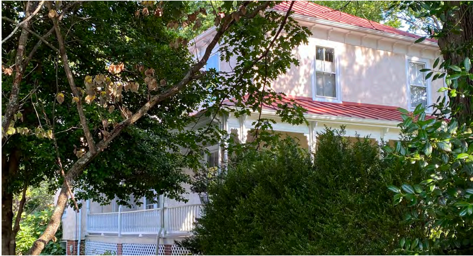
EXISTING CONDITIONS - SOUTHEAST
