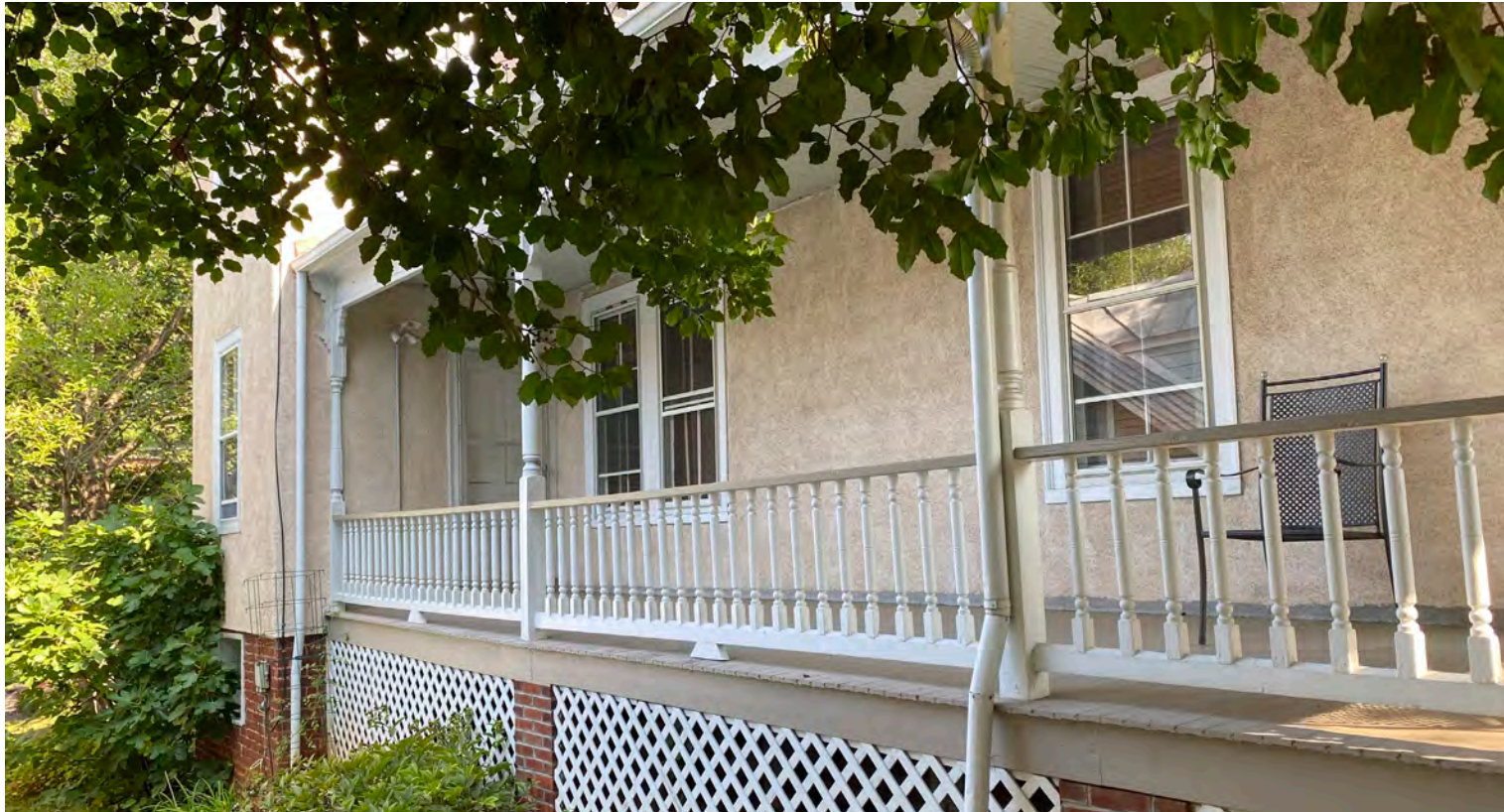
EXISTING CONDITIONS - SOUTHEAST
