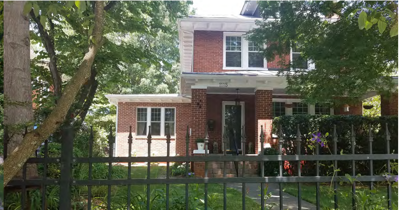
APPROVED ADDITION, COMPLETED
