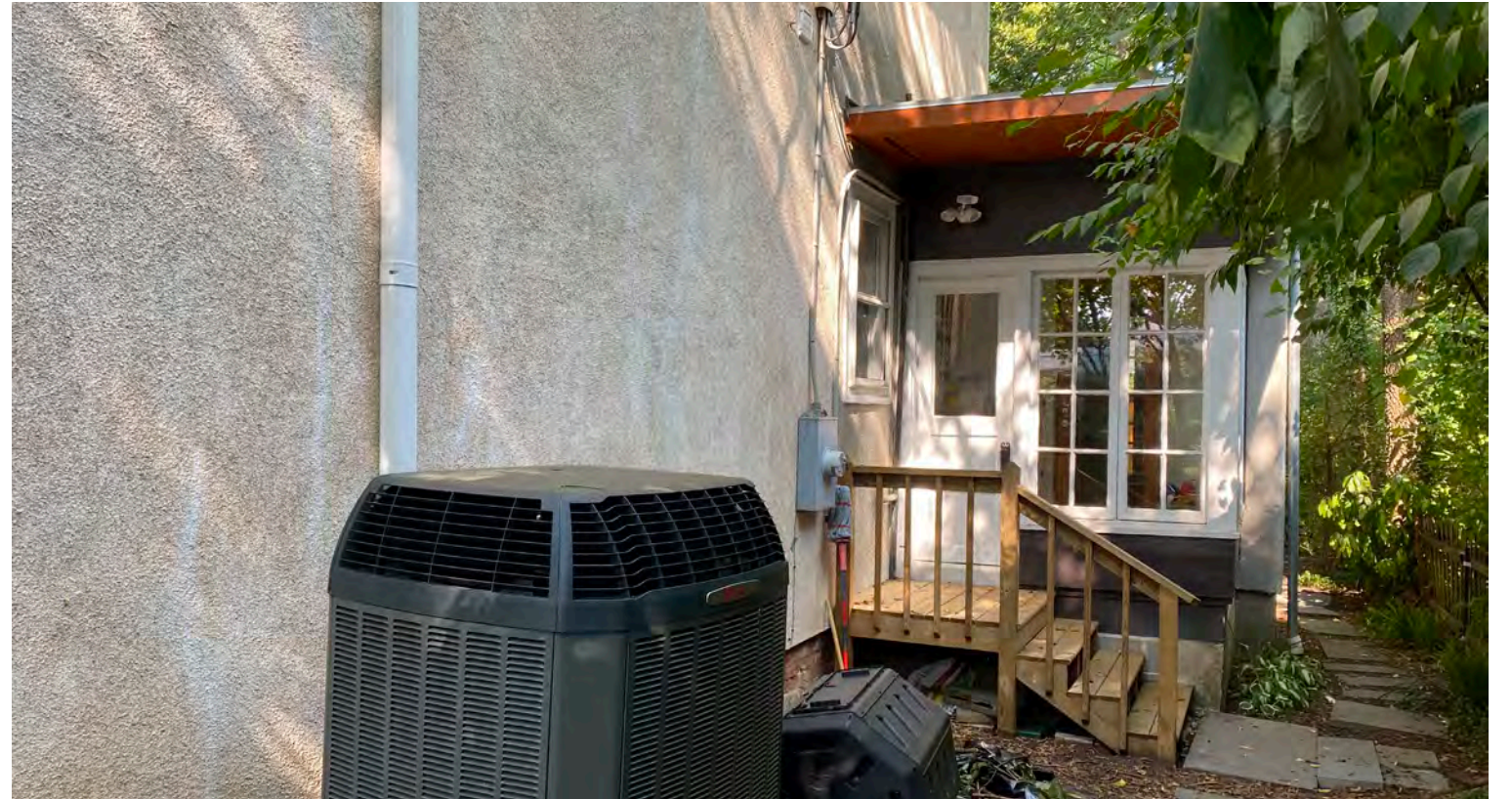
EXISTING CONDITIONS - NORTHEAST
