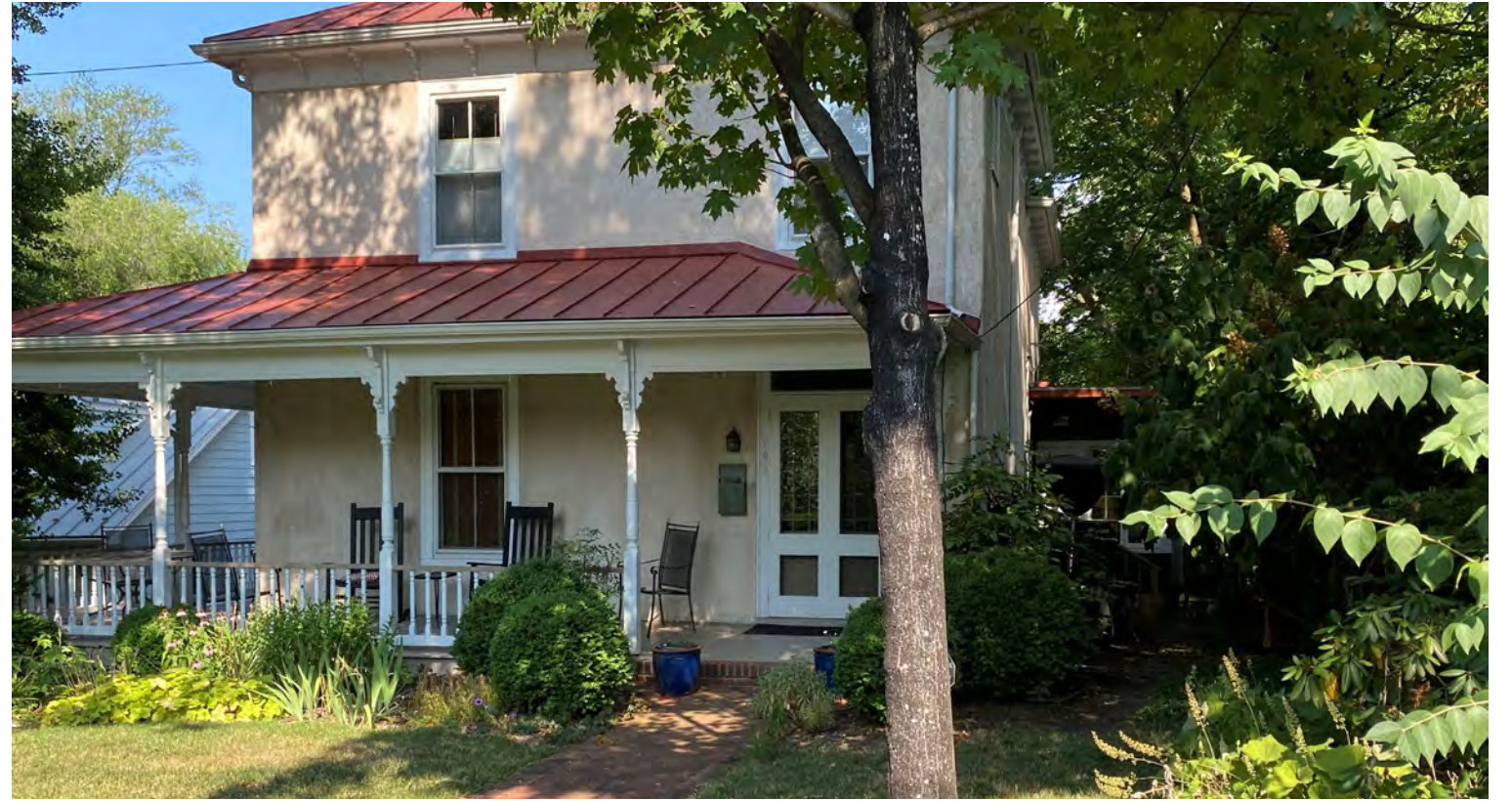
EXISTING CONDITIONS - NORTHEAST
