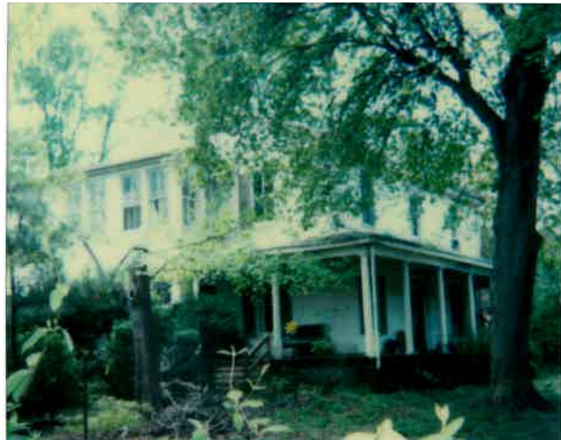
The property has been substantially altered over time. The enclosed sleeping porch on the left in these 2 images has been completely removed.
