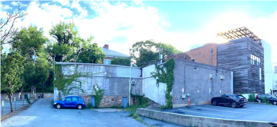
View looking north at south facade of 210 West Market Street
