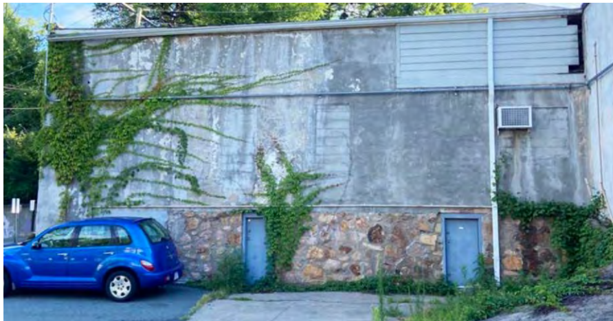
South elevation of 210 West Market Street
