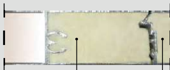
Polyurethane filled rails and stiles
