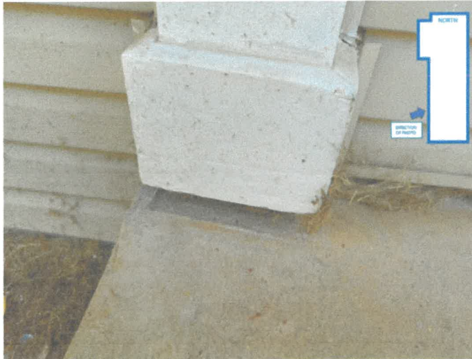
Photo 2: Imprints of the post in concrete indicate the slabs original position.
