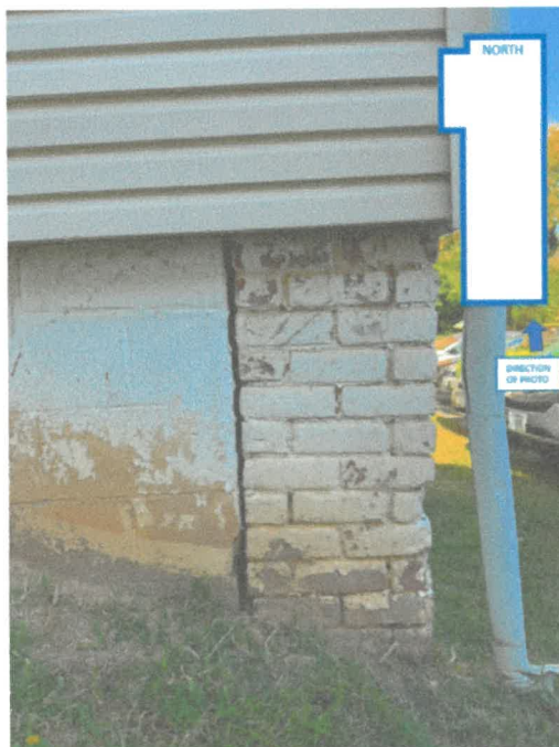
Photo 6: Perimeter piers with gaps between CMU infill and piers being larger at top.
