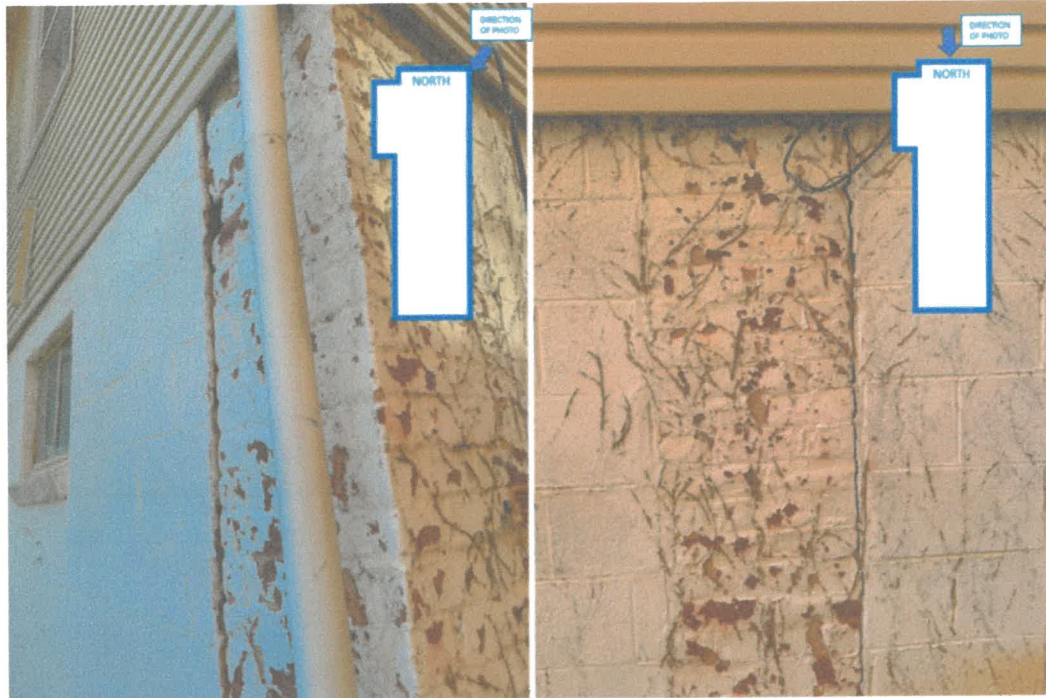
Photo 4/5: Perimeter piers with gaps between CMU infill and piers being larger at top.
