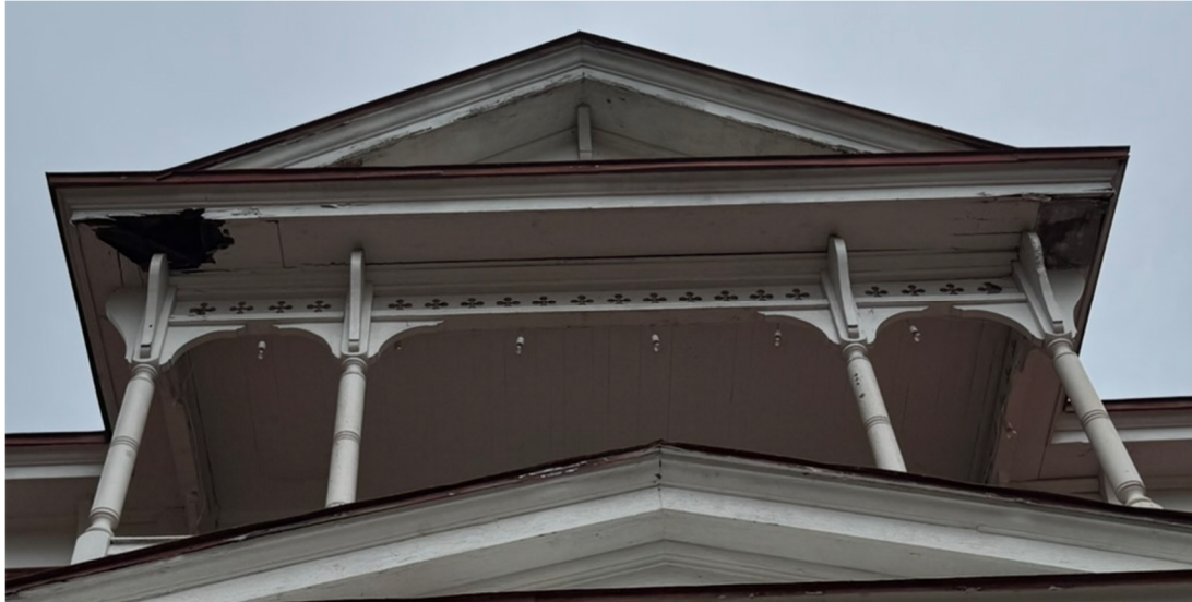
Photo 6: Front balcony with damaged soffit.
