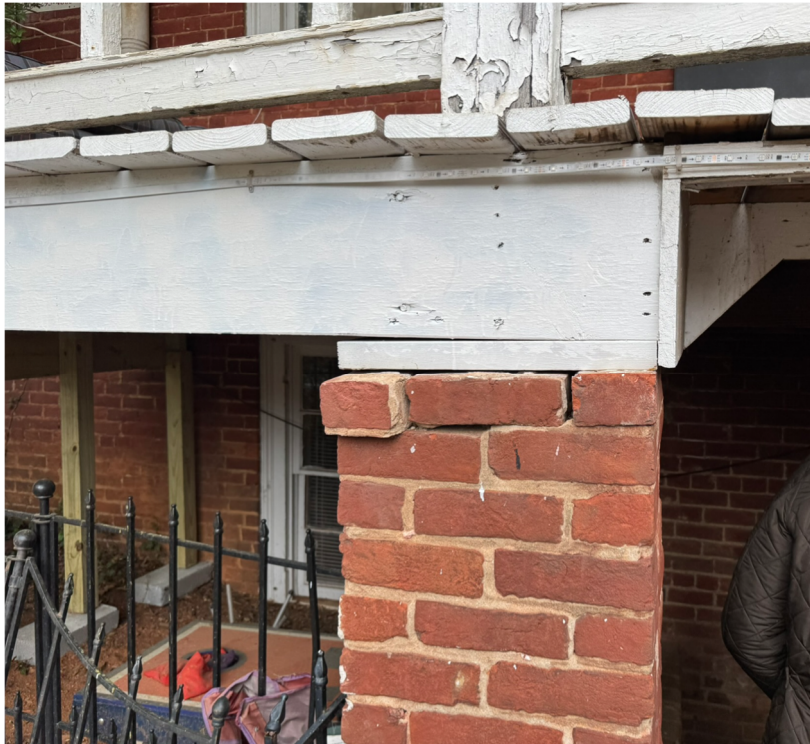
Photo 5: Front porch with wood posts and CMU foundations.
