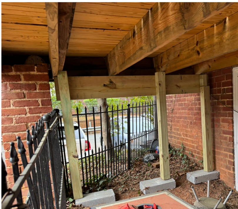
Photo 5: Front porch with wood posts and CMU foundations.
