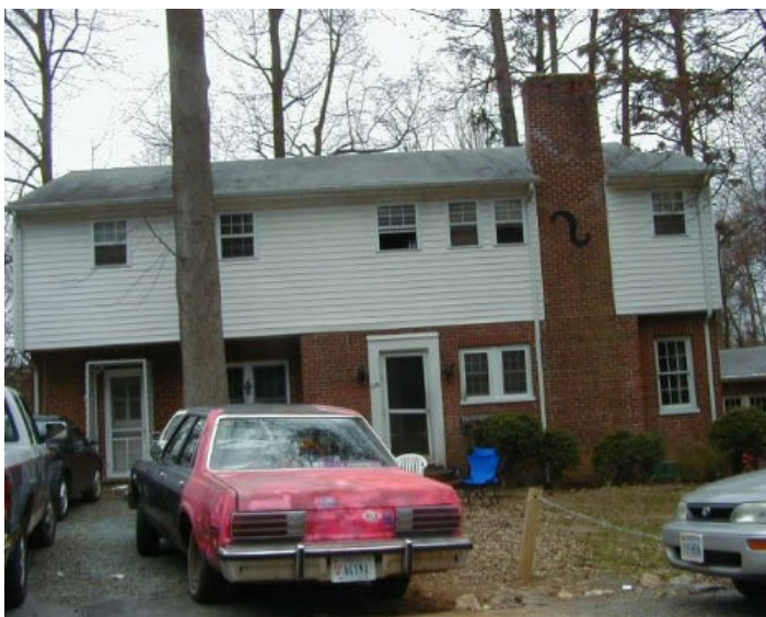
526 Valley Road (1935, altered)
