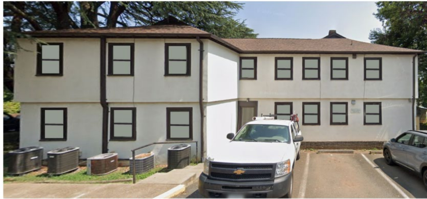
West elevation - Simulation of double-hung windows
